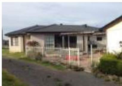
View of: Residential house Looking South Inspected on 12.09.2017
