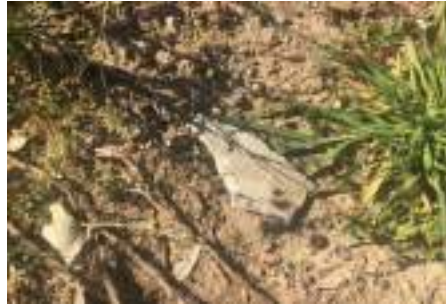
View of: Asbestos fragment in the south portion Looking South Inspected on 11.09.2017
