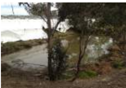
View of: Man made dam Looking west Inspected on 12.09.2017
