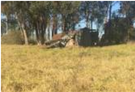
View of: Shed structures in the western portion Looking West Inspected on 11.09.2017
