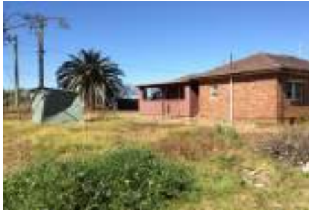
View of: Single-storey brick house and old shed structure in the front Looking South east Inspected on 11.09.2017
