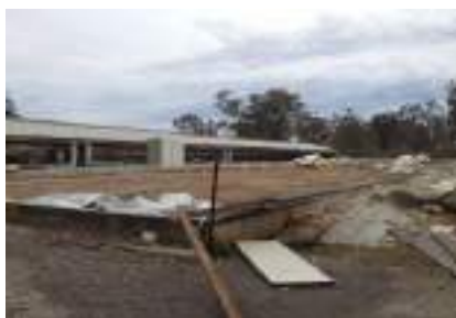
View of: Former poultry shed structures Looking West Inspected on 12.09.2017
