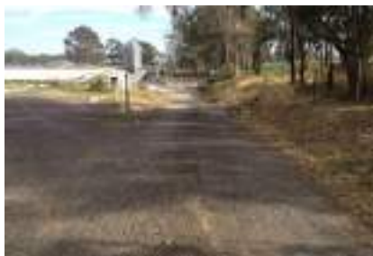
View of: Gravel & bitumen driveway Looking North Inspected on 12.09.2017
