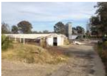
View of: Poultry shed structures Looking North Inspected on 12.09.2017
