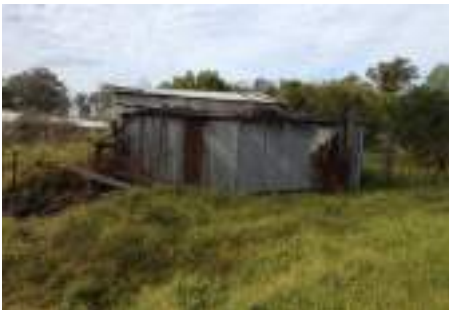
View of: Old metal shed structure Looking east Inspected on 12.09.2017
