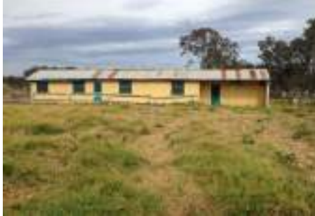
View of: Fibro building Looking east Inspected on 12.09.2017
