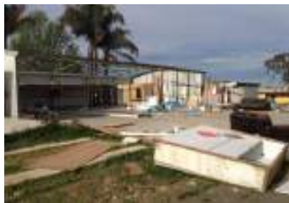
View of: Shed structures in the southern portion Looking South west Inspected on 12.09.2017
